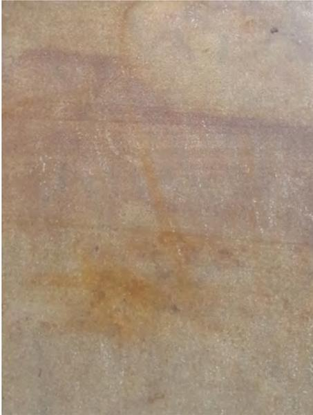
Fig. 2- Typical macroscopic feature of the Montjuïc Sandstone, including moderate evidence of lamination enhanced by the presence of Fe-rich minerals. Note the fade of oxidation, a common feature in this rock when it has undergone severe acid cleaning (façade of Passatge de la Pau street, Barri Gòtic, Barcelona).
