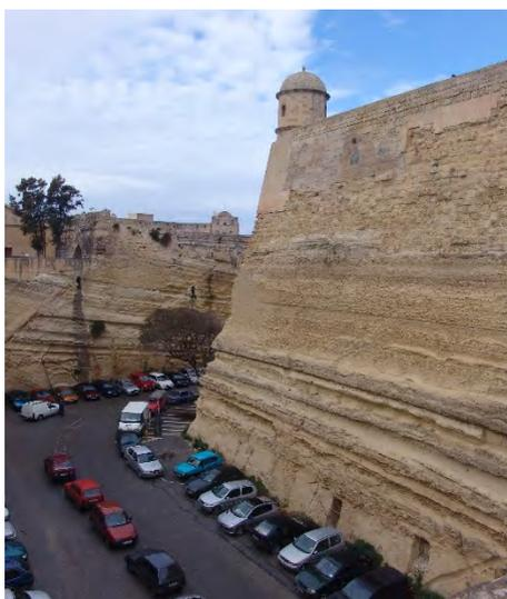
Fig. 7- Valletta, Malta. Rock bench and masonry degradation (Marta Acierno 2011).
