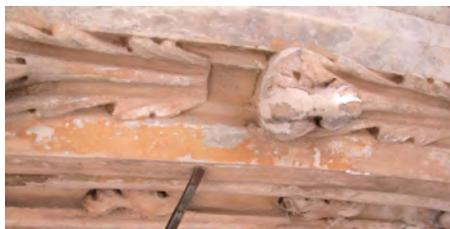
Fig. 5- Detail of the Siena Cathedral main façade. Overlapping of the two films on marble (yellowish the first type, greyish the second type).
