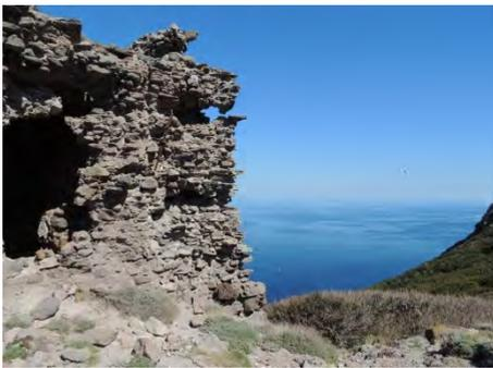
Fig.7 - Tower of Barbici: the deeply eroded masonry.
