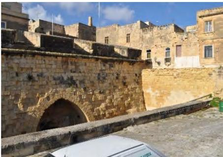
Fig. 8- Birgu, Malta. Scaling and back weathering on southern fronts (M.Acierno 2011).
