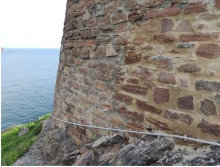
Fig. 5- Tower of Porto: the restored surface.
