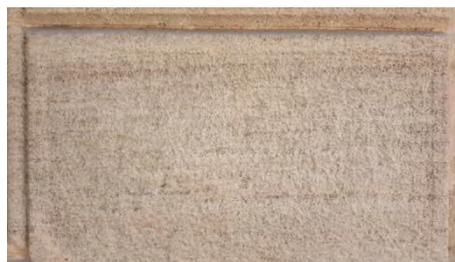
Fig. 1- Typical macroscopic feature of the Montjuïc Sandstone, including moderate evidence of lamination and cross-bedding after diagenetic lithification and pervasive silicicementation (façade of Passatge de la Pau, Barcelona).
