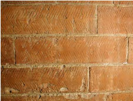
Fig. 8- Siena Town Hall. Herringbone bricks at the first floor of the main façade.
