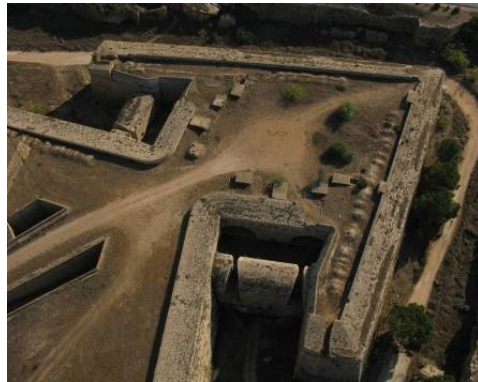
Fig. 1- Martinengo Bastion (Eppich, 2015)
