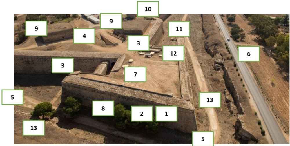
Fig. 3- Martinengo Bastion during conservation (UNDP, 2016)
