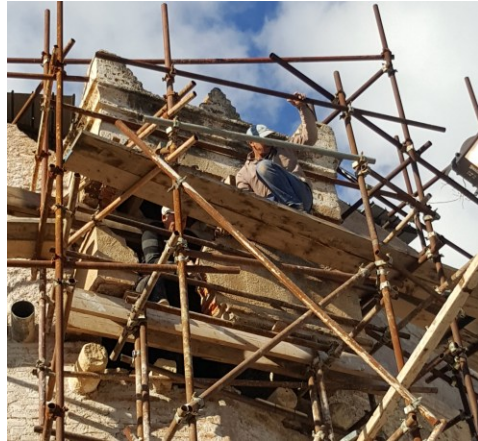
Fig. 8- Restoration of the observation tower
