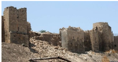
Fig. 8- Destruction of western wall of the citadel (Orient, 2014)
