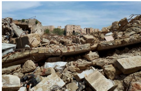
Fig. 9- Destruction around the citadel (SANA, 2016)
