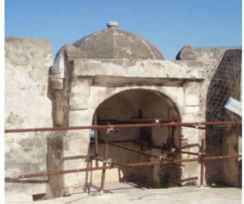
Fig. 4- View of the ribbed dome
