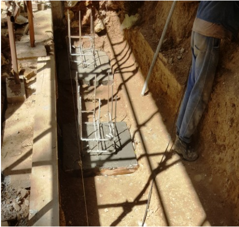
Fig. 6- Consolidation of the gallery
