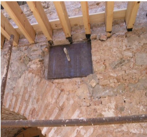
Fig.7- Consolidation of the vault
