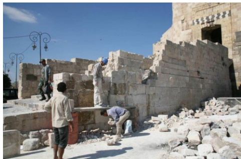
Fig. 10- Restoration of the citadel entrance (DGAM October, 2017) 5
