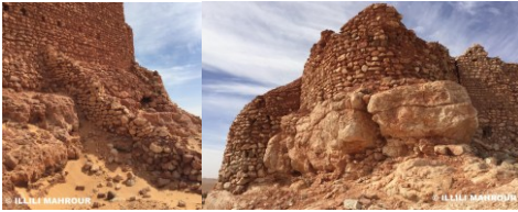
Fig.15-Northern circular tower and stone buttresses, Bousaïd - Si Abdelaziz fortress, Semjane (Mahrou, 2018)
