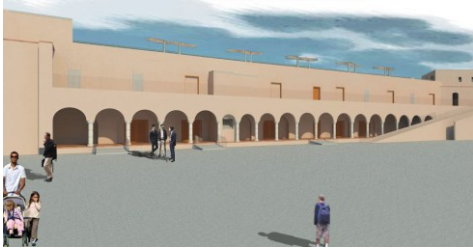
Fig. 9- General view of the project after intervention
