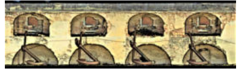
Fig. 15- Orthophoto detail of the city wall regarding the military lodgings on the ground floor and the firearm openings on the upper level (graphic elaboration by A. Altadonna)
