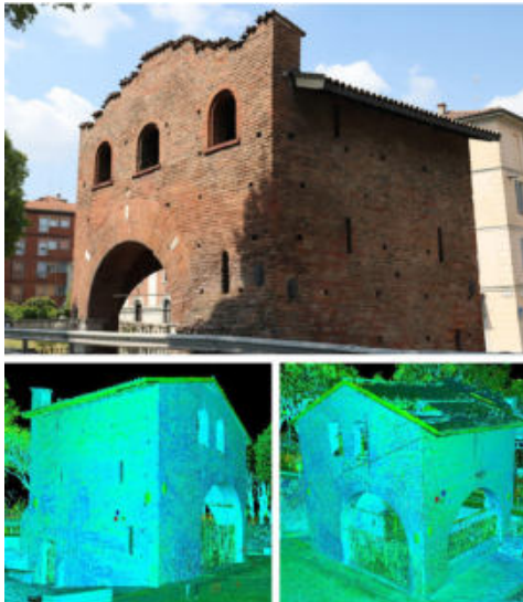
Fig. 4- Porta Nuova in Pavia. High resolution point cloud (1-3mm) from Terrestrial Laser Scanner survey (Raffaella De Marco, 2021)
