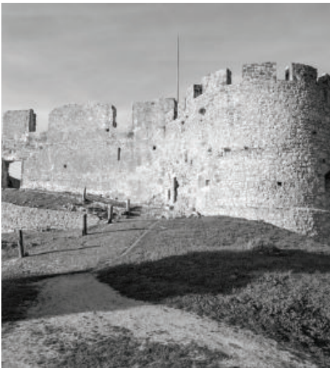
Fig. 3- Castle of Torres Vedras, view of the south elevation of the castle (photo by Fabiana Guerriero, 2021)
