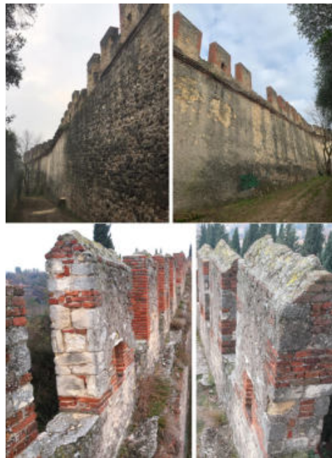
Fig. 2- Views on present state of conservation and restoration traces of the mediaeval walls (2020)
