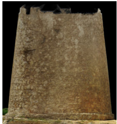
Fig. 6- Front of the tower in orthographic projection, retouched point cloud with photographic colour mapping (Verdiani, 2022)
