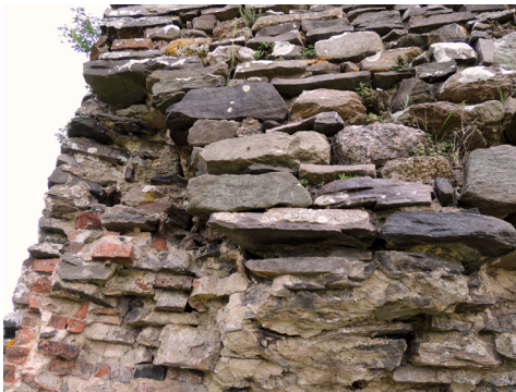
Fig. 6- The small, roughly hewn ashlar of grey to green-purple quartzite constituting most part of the perimeter walls (photo by Fabio Fratini, 2022)
