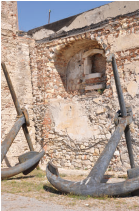
Fig. 14- Detail connections between the Fort Campana and city wall enclosures at north (picture by the authors 2021)
