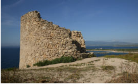
Fig. 1- View of the Tower (photo by Verdiani, 2022)
