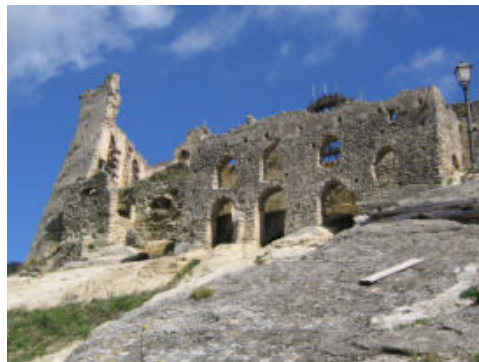
Fig. 10- Arched wall structures (photo by Caterina Gattuso, 2011)
