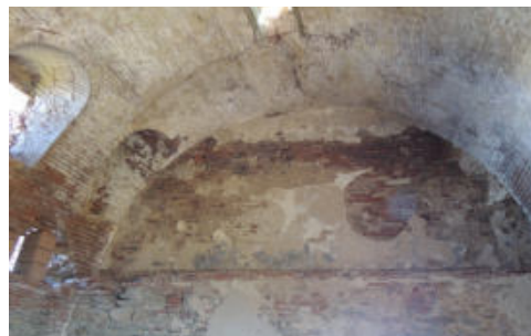
Fig. 3- Room with a barrel-vaulted roof at the apex of which is present a square trapdoor (photo by Fabio Fratini, 2021)
