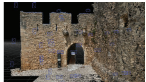
Fig. 7- Castle of Torres Vedras, entrance to the fortified complex, view of the dense point cloud, obtained through the process of aerial photogrammetry and identification of the acquisition points (Fabiana Guerriero, 2021)
